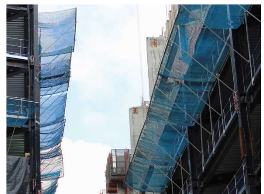
Fixed Catch Platform installation
